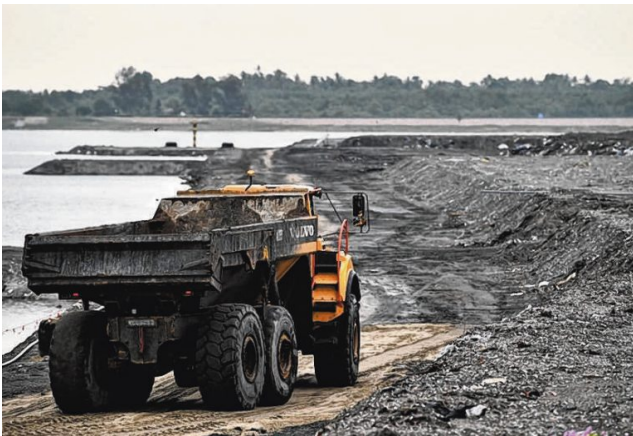
The 350ha Semakau landfill, which can hold 28 million cubic m of waste, is expected to reach full capacity by 2035. A study is under way to determine if waste there could be used as an alternative fill material. ST PHOTO: LIM YAOHUI
